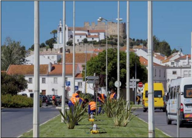
Figure 5 Equipment deployment in a very busy urban setting utilizing available geophone planting sites between roads.
